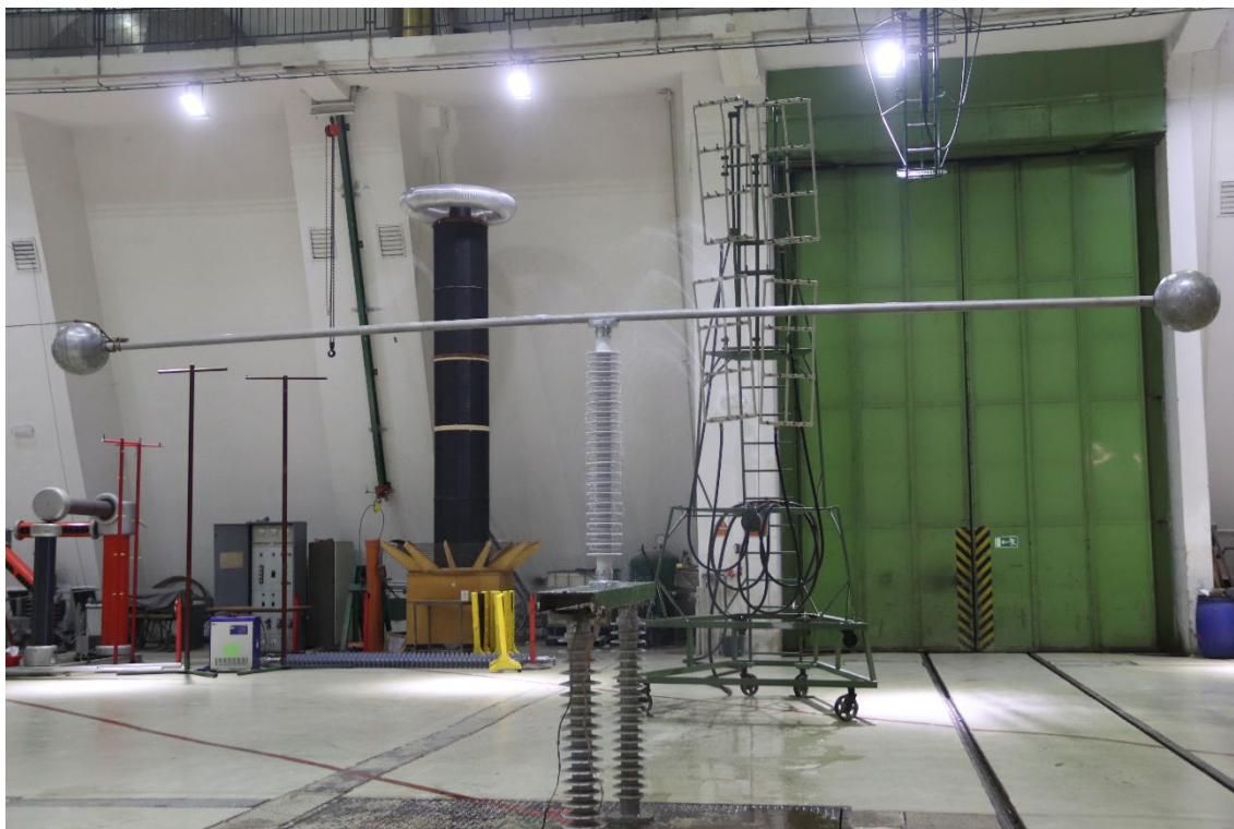
Figure 5 Test arrangement during the low-frequency voltage wet withstand test
